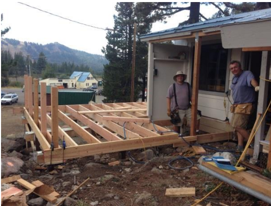
Framing the new deck
